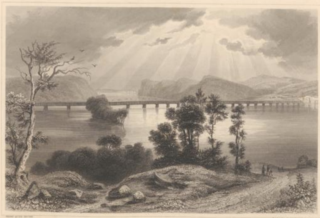
COLUMBIA BRIDGE (SUSQUEHANNA)
