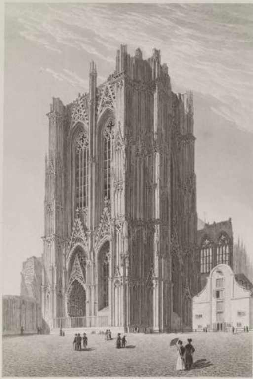
View of the Westwerk
